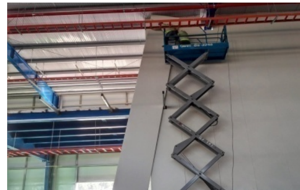
Lắp dựng vách panel Installation of wall panels
