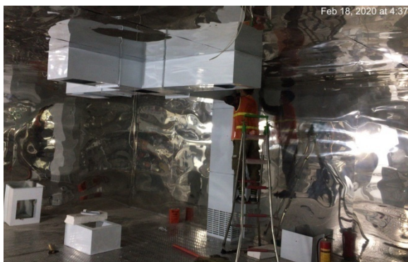
Thi công kho sấy lạnh Installation of drying room
