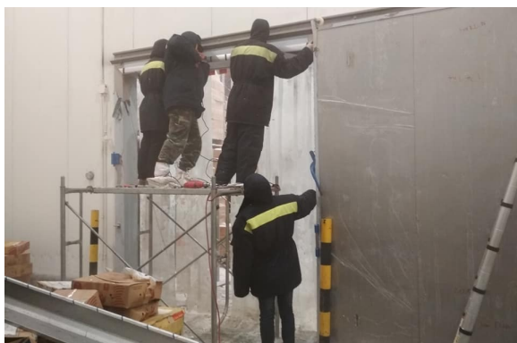
Lắp cửa kho lạnh Install cold storage door
